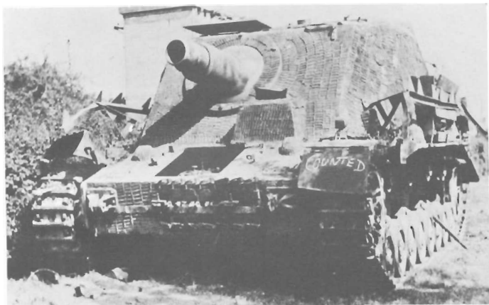
Counted as war booty, this "Sturmpanzer" was captured by the Allied in Italy in 1944. Note the driver compartment is without visor.
