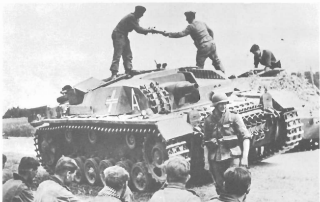
Sturmgeschuetz III, Ausf. B, being resupplied in France, 1940. Hatches in top of superstructure are the only access for crew. However, emergency exits were provided for driver and radio operator through openings in the top plate of the front hull armor.
