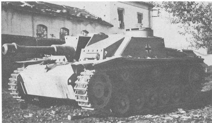
An abandoned assault howitzer in 1944. Note the bolting of the additional 30 mm armor to the front of the vehicle.
